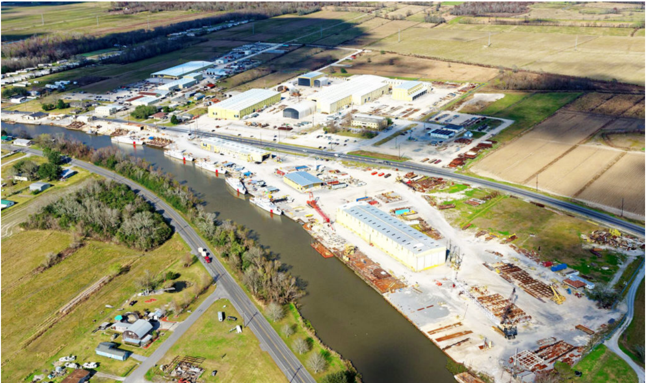
Aerial image of Bollinger's shipyard at Lockport,
