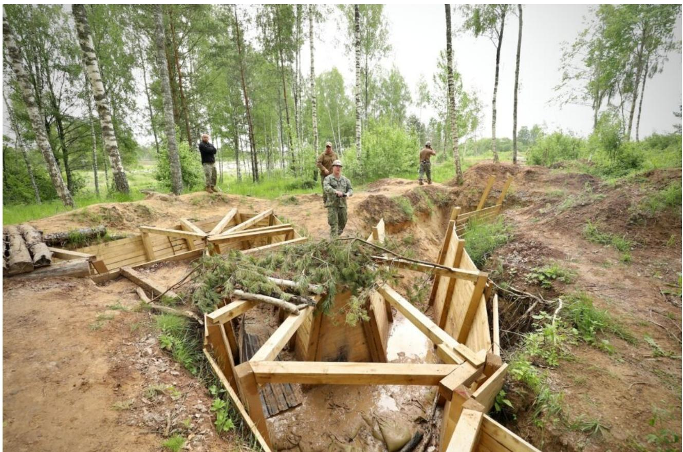
U.S. Navy Sailors assigned to Naval Construction Battalion 14 and Marines assigned to 8th Engineering Support Battalion conduct trench reinforcement training to increase combat engineering capabilities during exercise Baltic Operations 2025 (BALTOPS 25), June 6, 2025, in Skrunda, Latvia.
